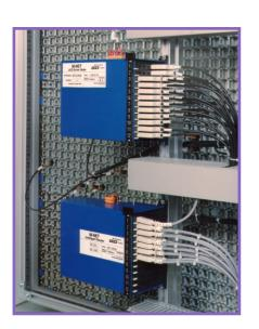
LEDs or LED modules - connect to the M-Net LED driver node using standard plug and cable sets. These cables can provide either single or multi-function/colour LED connections.
